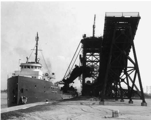
Sandusky, Ohio. Coal docks. Loading coal into a lake freighter at the Penn. R.R. No. 3 dock. May 1943
